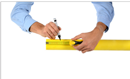
4. Medir la zona a rascar. Measure the scraping zone.
